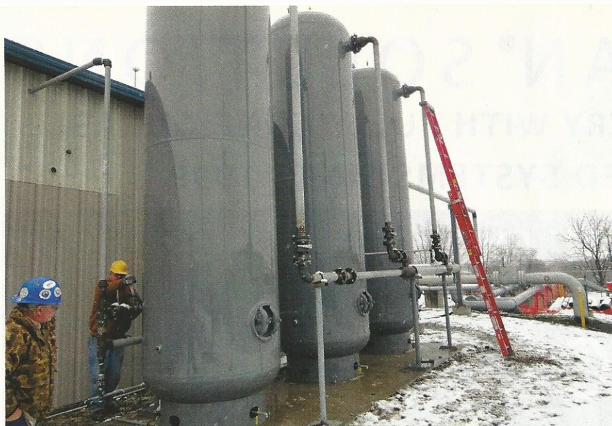
■ The starting air compressors supply three 2560 gal. (9691 L), 200 psig (13.8 bar) air receivers installed outside the compressor building.
